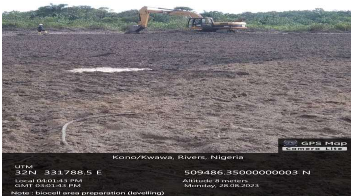
Plate 1: Bio-Cell Levelling
